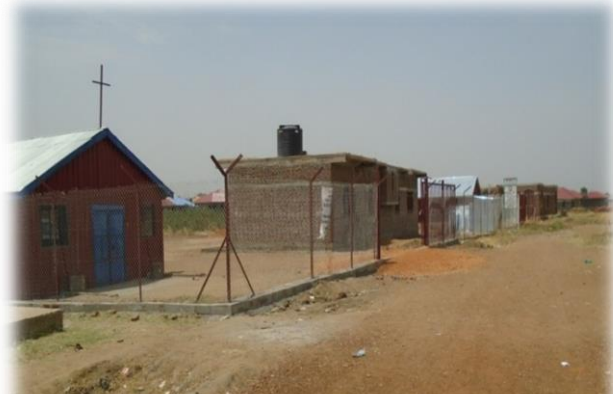
Bethel SRC new erected fence at Mangateen
